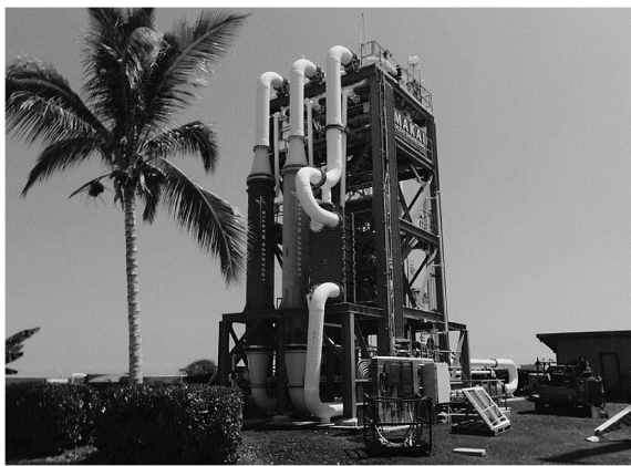
Fig. 8 100 kW OTEC pilot plant in Big Island, Hawaii
